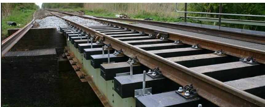
Fig. 8: Waste Management for Construction of Railway Tracks [25].
